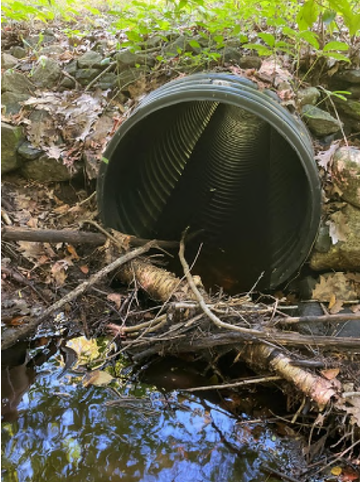
Figure B-49 Exit of Wilson Hill Road Culvert
