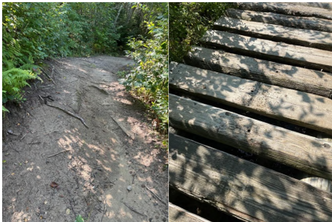
Figure B-12 Erosion on Existing Skid/ATV Trails (L) and Evidence of Snowmobile Use on Bridge (R)
