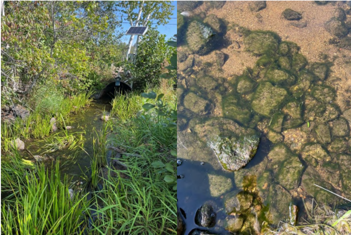
Figure B-25 Townsend Brook Downstream of Lake Shore Drive Culvert
