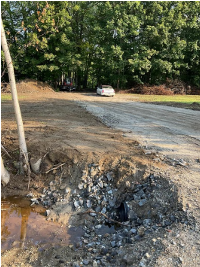
Figure B-61 Construction on Hathaway Road
