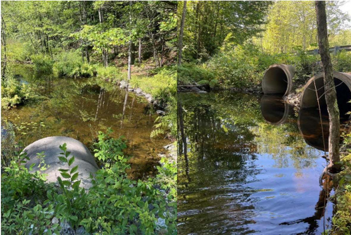
Figure B-45 Armored Inlet (L) and Outlet (R) of the Culvert at the Little Wilson Pond Outlet
