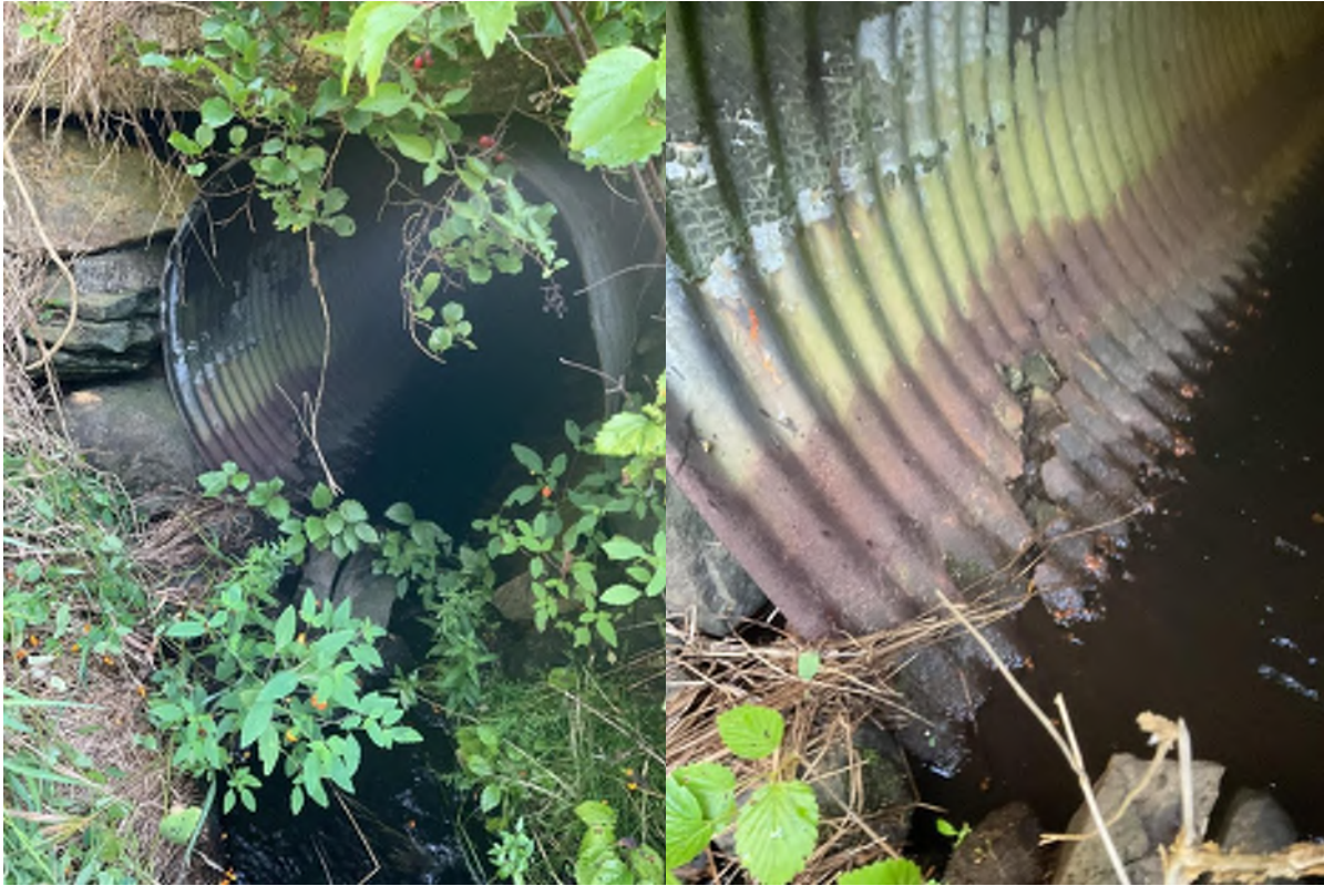
Figure B-59 Summer Street Culvert
