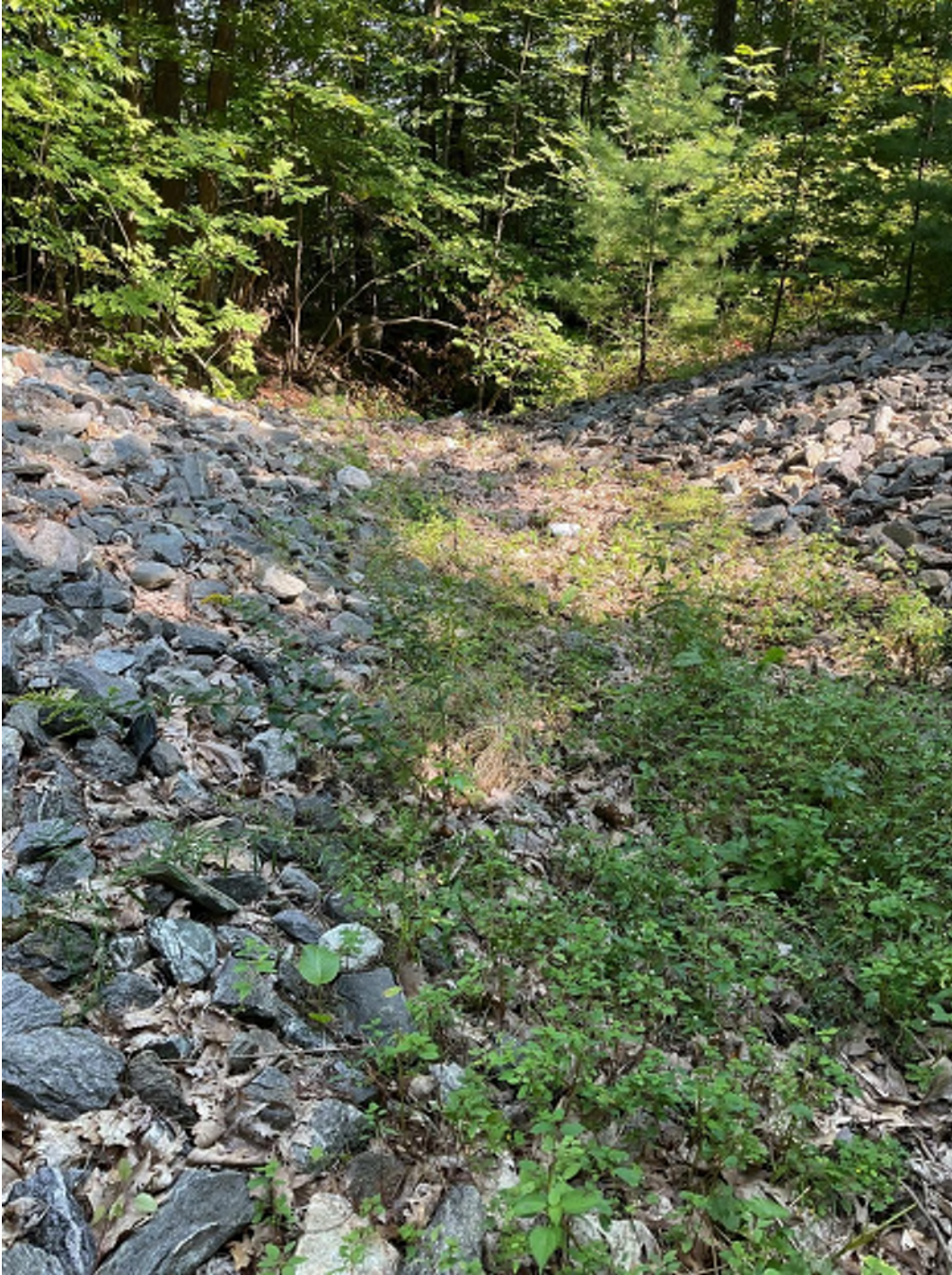
Figure B-42 Lunn Rd Culvert Replaced with Riprap
