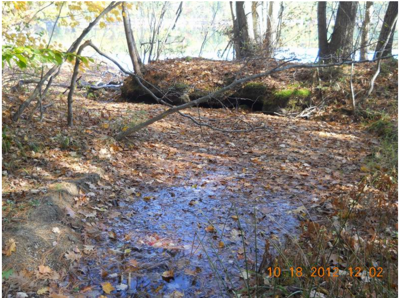
Outlet delta filled with sediment and leaves. Note the apparent high flow erosion around base of the trees
