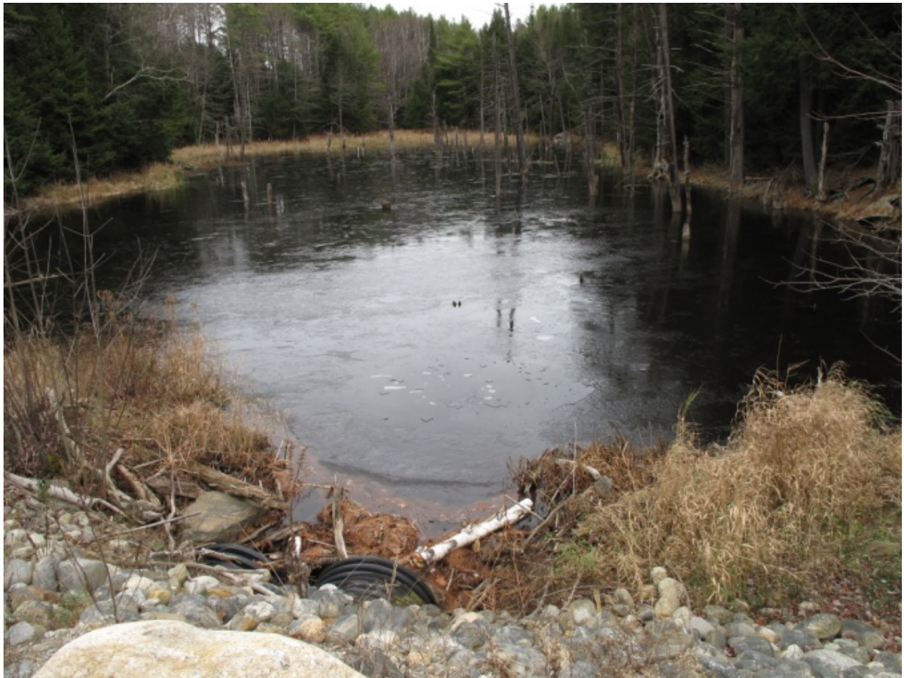
Wetland pond near operational sandpit. Sticks and debris has partially dammed the outlet
