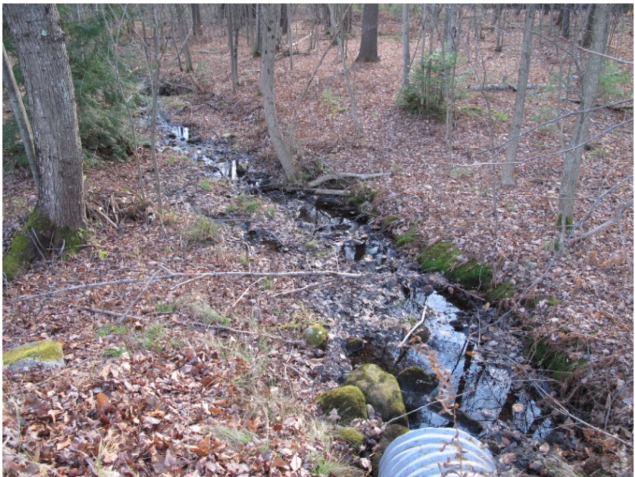
Moderate roadside slope causing some minor channeling and erosion problems. Outlets to a small wetland
