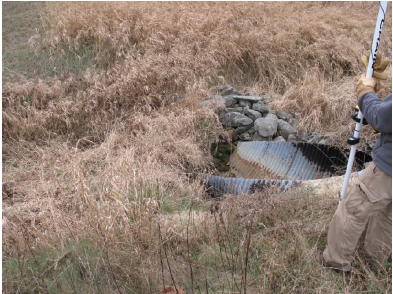
6 ft diameter inlet culvert shown. Two major drainage channels for the area converge here
