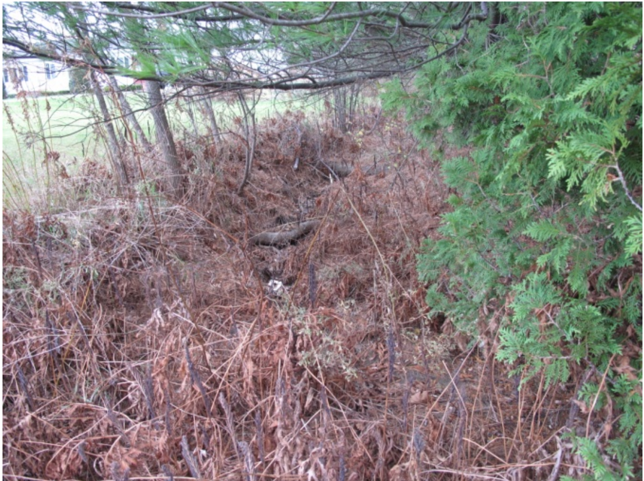
Runoff channel down moderate slope. Outlets to steep shoreline with evidence of a sediment delta
