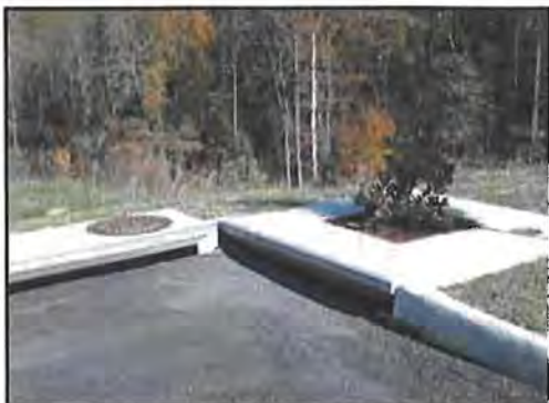
1. Inspection of Filterra and surrounding area
