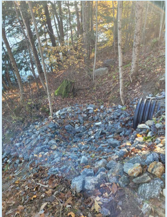
A new plastic culvert leading to an outlet with riprap.
